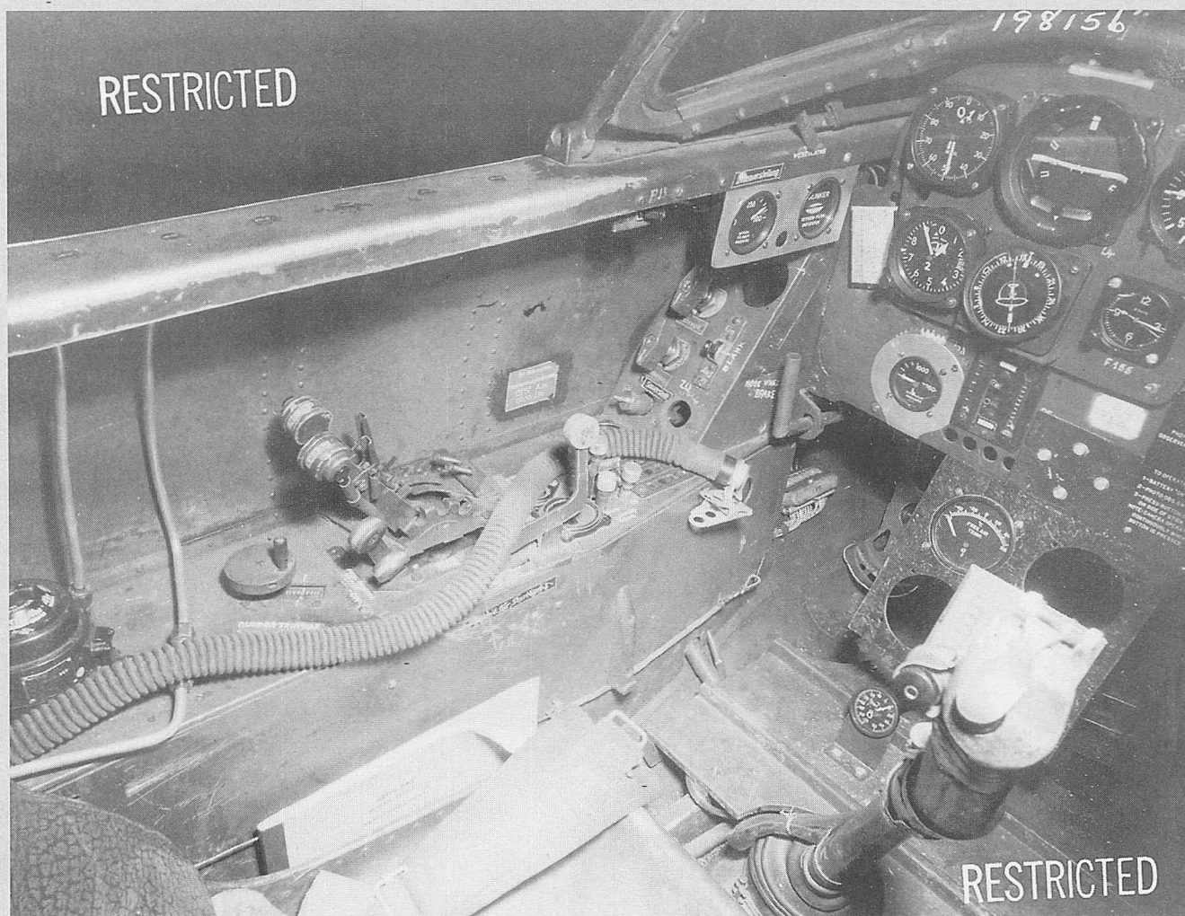
This photograph was used to document the Me 262 in a December 1945 report on foreign equipment. This shot illustrates the left auxiliary console that contains the throttles, and flap and landing gear switches and indicators. (Air Force Museum Collection)
