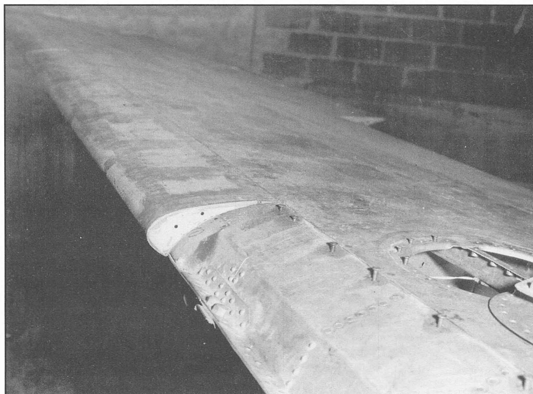
The starboard leading edge slots in the retracted position. The slots were fully automatic in the operation, the position being determined simply by aerodynamic forces upon the wing. (Air Force Museum Collection)
